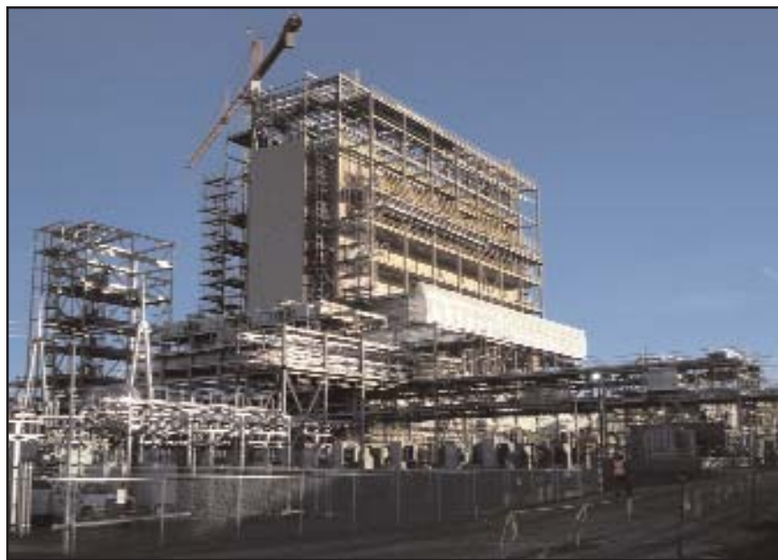
■ Figure 1. Renewable Energy Corp.'s new plant in Moses Lake, WA, will use a fluidized-bed process to produce polysilicon, using trichlorosilane as the carrier gas. Photo courtesy of Fluor Corp.
